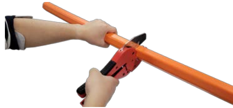
Duct Cut by Cutter
