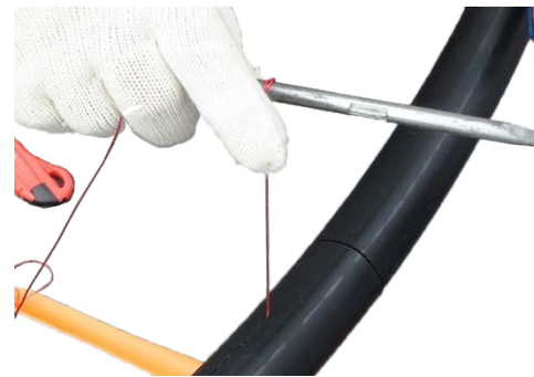
Cut 2nd sheath by rip cord (if exist)
